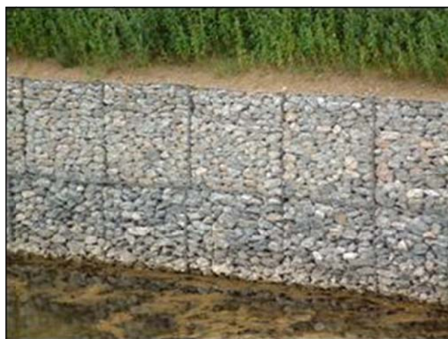
Visually unsightly stone filled gabion baskets.
