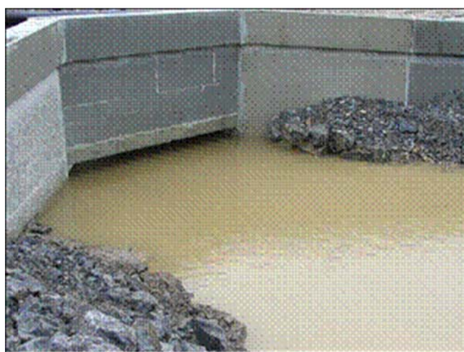
Is the culvert adequately sized?
