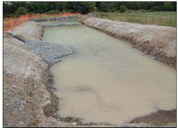
Silt control pond. Note hose conveying pumped silt laden waters with its outlet positioned within the gravel mound thus ensuring no disturbance of pond contents.
