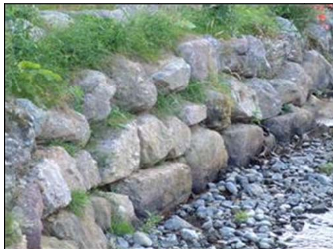
Revegetation of rock armour facilitated by the placing of locally sourced topsoil (to ensure no importation of non local grasses and shrubs) between each layer or course of boulders at installation time.
